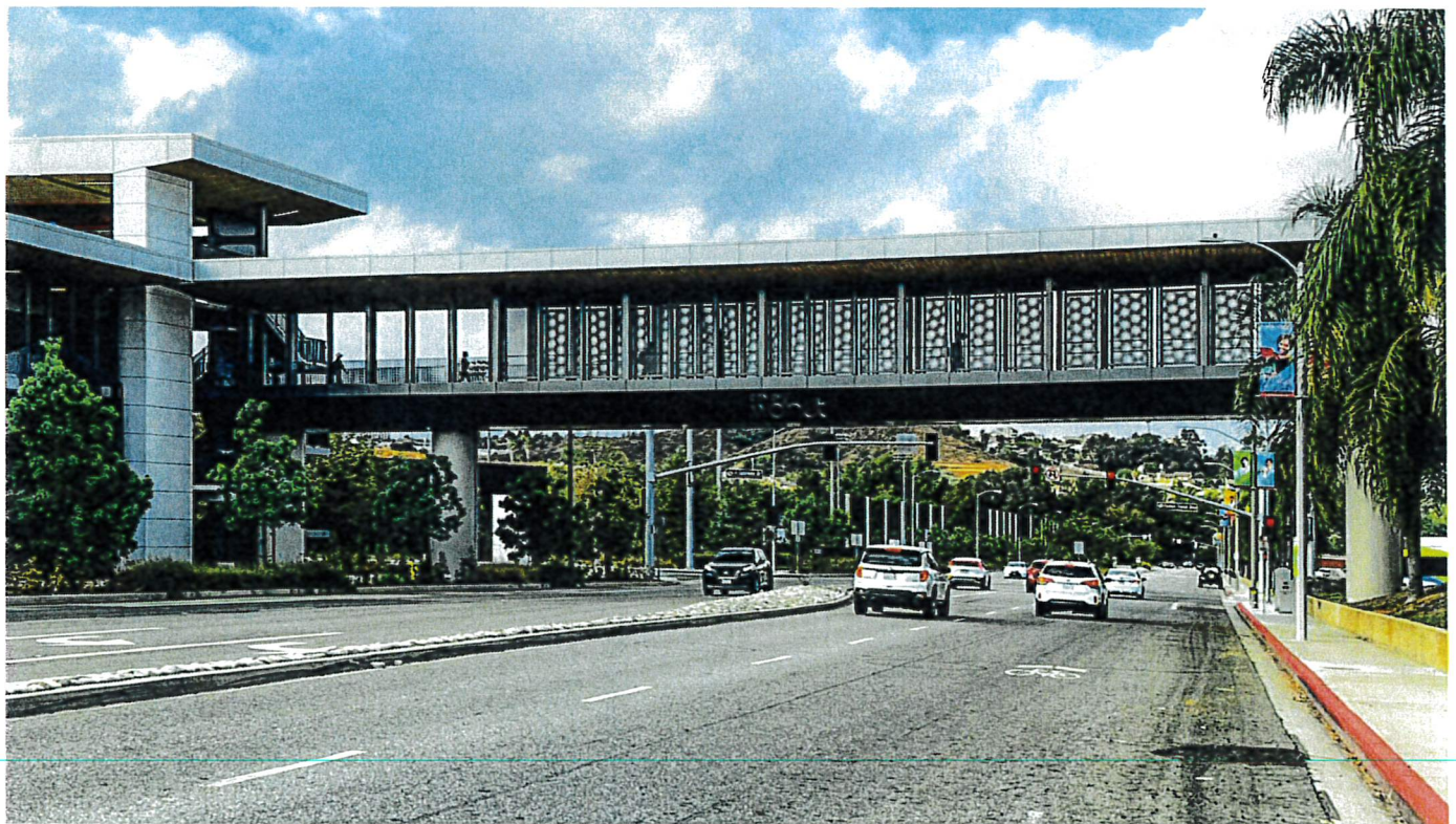
Bridge Signage - Photograph looking west on Temple Ave near Bonita Ave.
