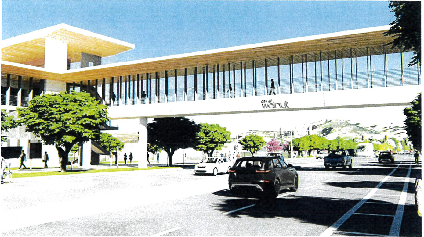
Bridge Signage - View looking west on Temple Ave near Bonita Ave.
