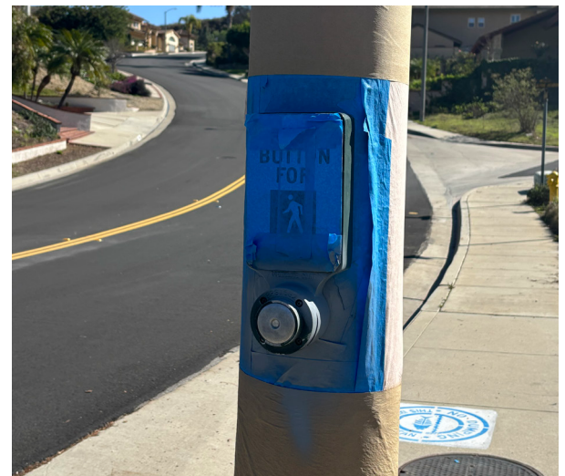
Lights being repainted
