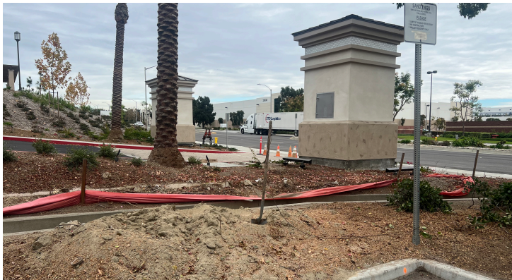
Sandbag area located at 21701 Valley Blvd.
